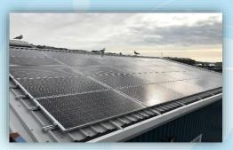
Solar panel with 50 kW capacity
